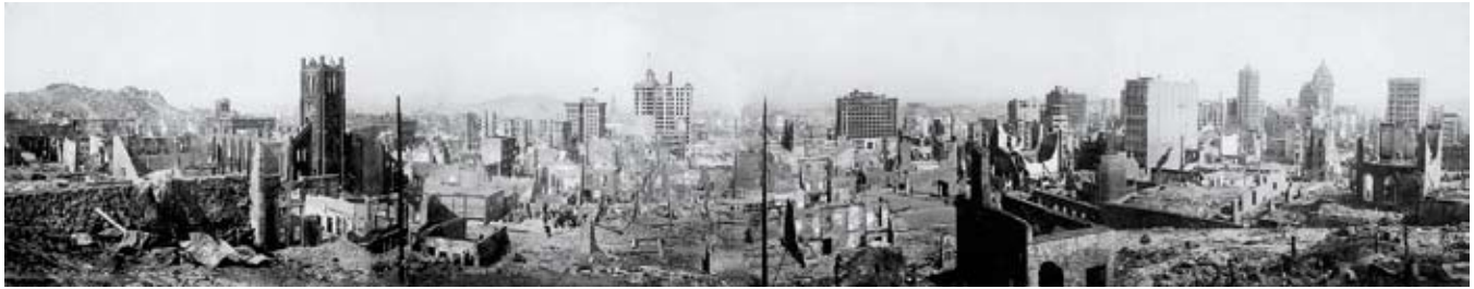
View of damage from the San Francisco earthquake of 1906.
