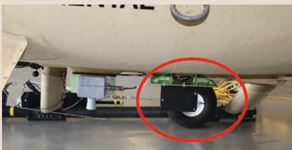
Laser micrometer installation
