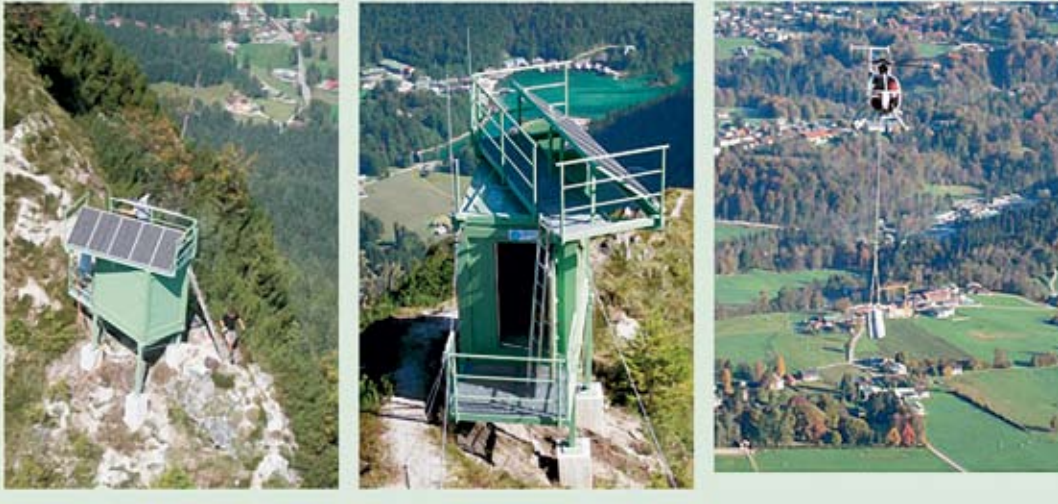
Transmit station at Gruenstein mountain and helicopter transport of GTS transmitter rack
