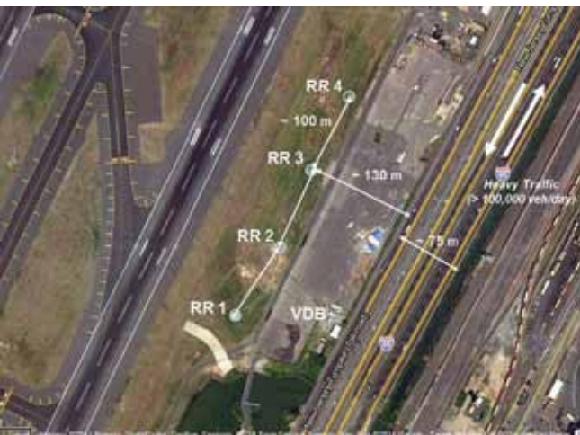
FIGURE 8 LAAS Ground Facility site at Newark Airport showing GBAS antenna locations
