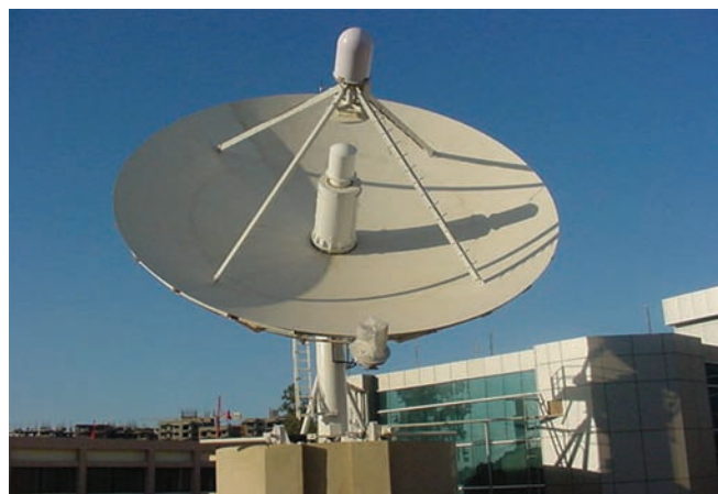
11 meter C-band uplink antenna at Bangalore
