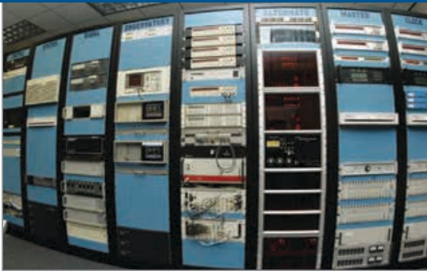
The U.S. Naval Observatory Alternate Master Clock at 2nd Space Operations Squadron, Schriever AFB in Colorado. This photo was taken in January, 2006 during the addition of a leap second. The USNO master clocks monitor GPS timing.
